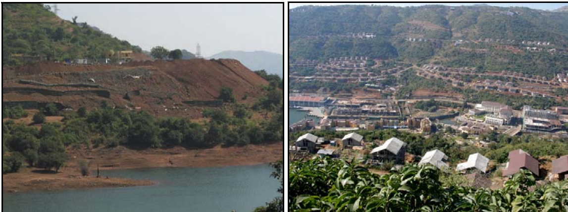
Construction in Hills - Lavasa
