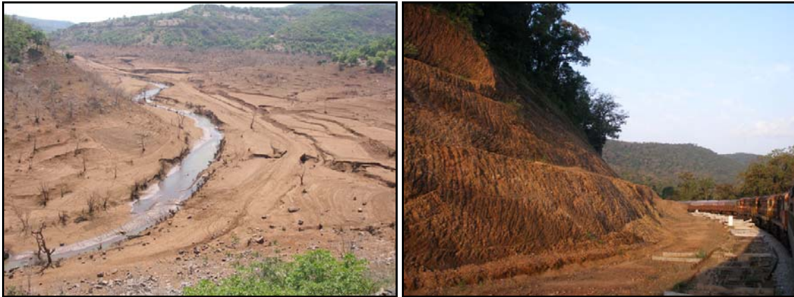
Area inundated under backwater & cutting of hills for Rails
